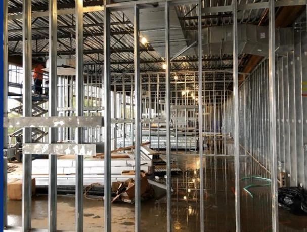
Interior wall framing in progress on 3<sup>rd</sup> level
