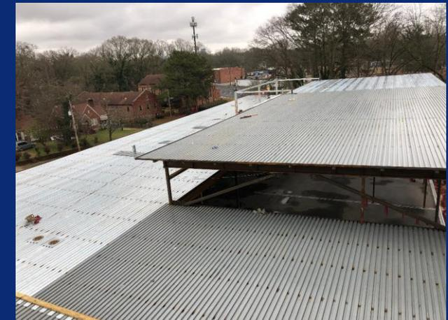
Decking for 2<sup>nd</sup> floor roof and stem lab pop-up installed
