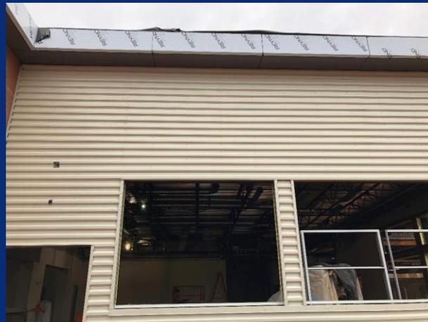
Metal panels, soffits and storefronts installing on south elevation
